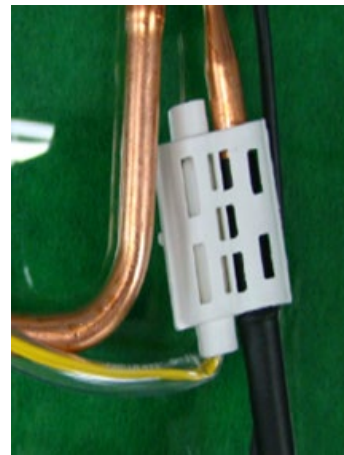
Sensor facing left (correct)
