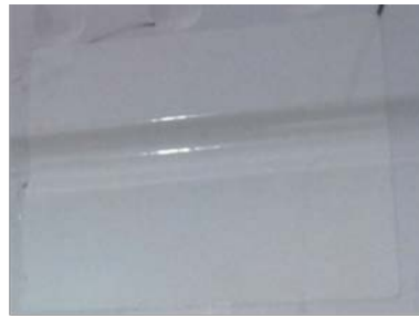
#5 Paste a label sticker on the crack area
