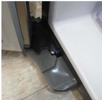
Hinge Cover Installed
